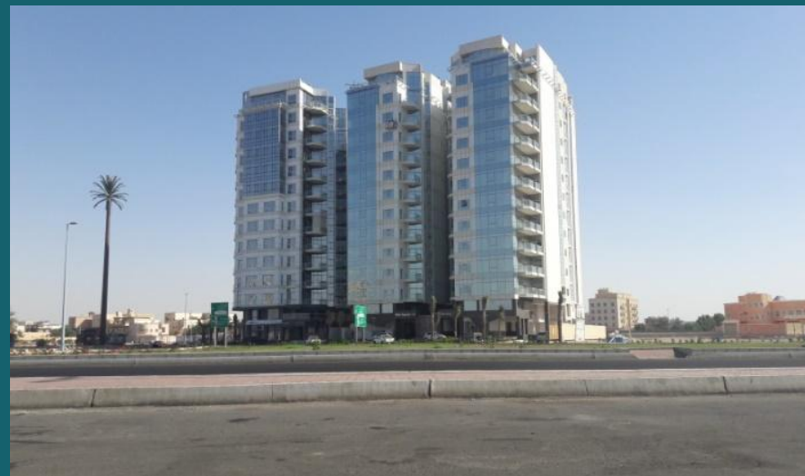
Obhor Residence 1&2 Location: Jeddah
