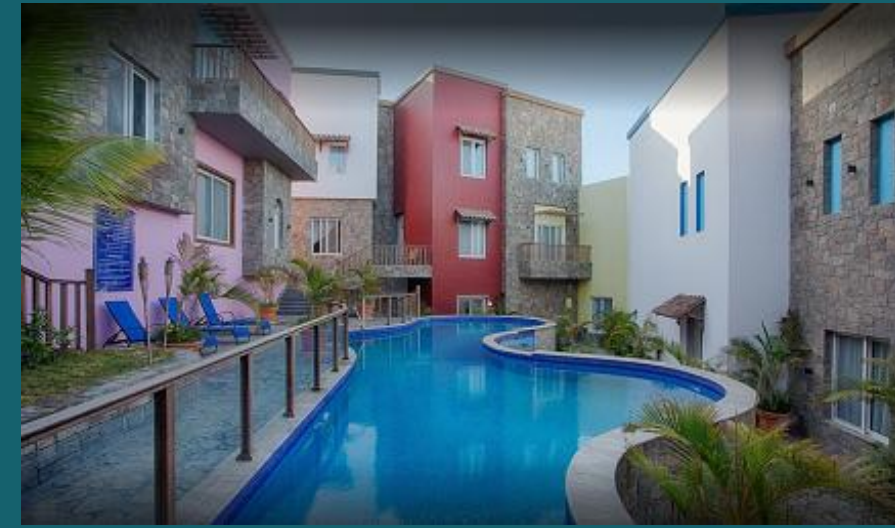
Desert Home Resort Location: Jeddah
