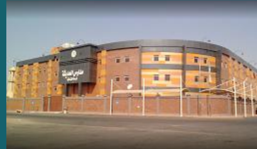
Al-Haditha International School Location: Yanbu
